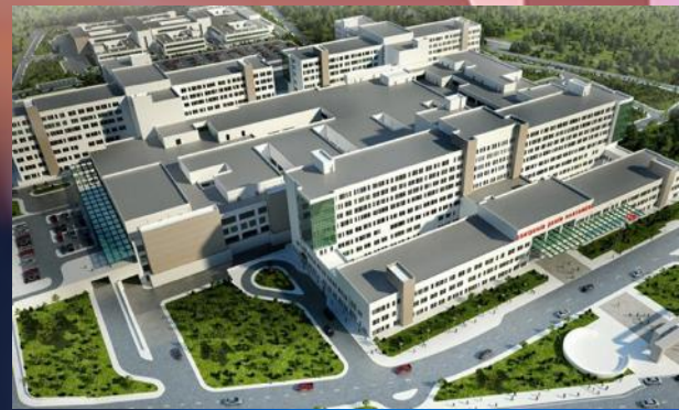
Eskişehir Integrated Health Campus 1080 Bed Capacity
